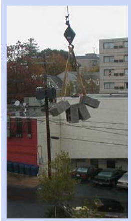
Twenty-four bricks were lifted to the roof for the setup of the satellite dish
